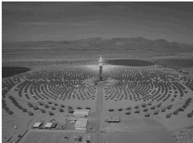
Figure 6: Solar tower with glass mirrors. (National Workshop on "Solar Thermal Power Generation" at IIT Bombay April 28, 2008)
